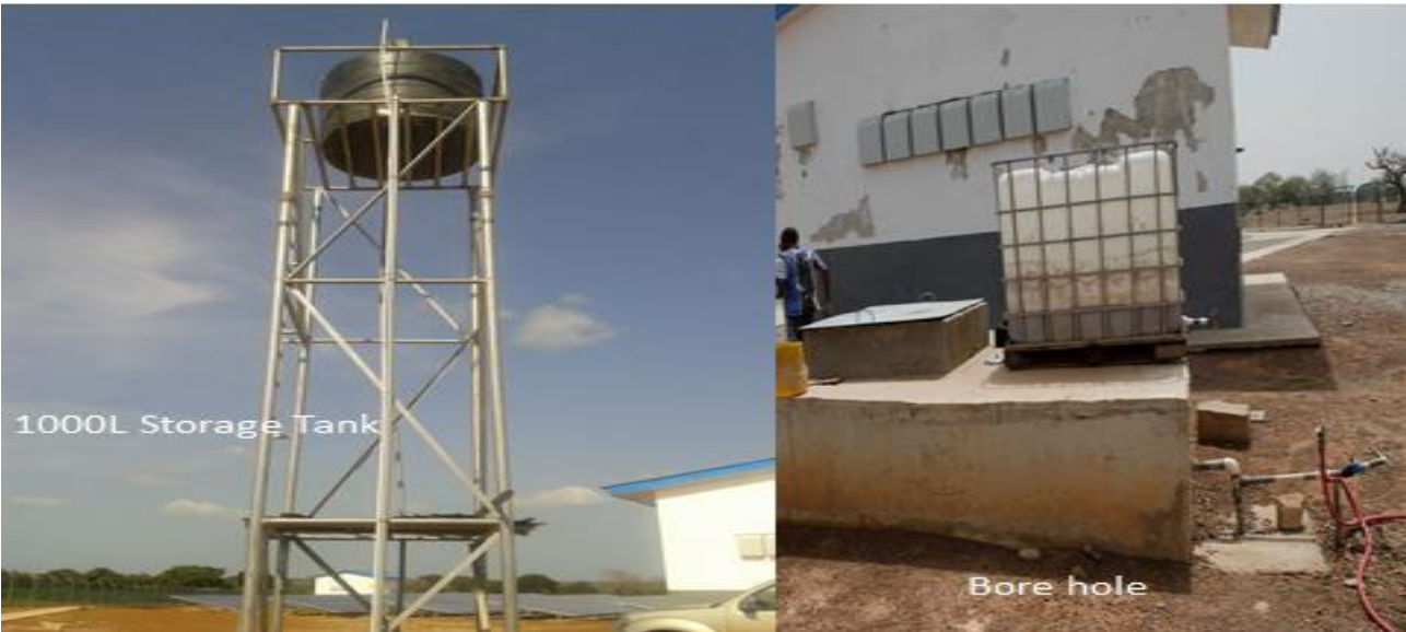
Plate 3-2: Borehole & Storage Tank for Water supply at Navrongo PV Power Plant
