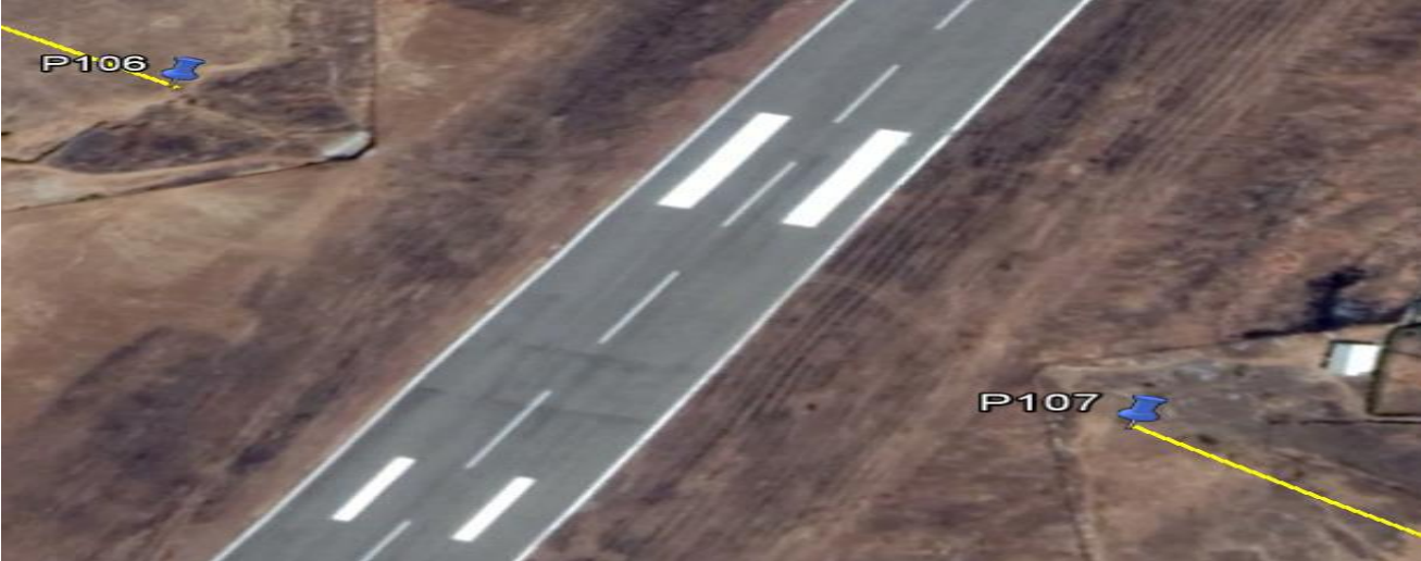
Plate 3-1: Area under Wa-Airstrip for overhead interconnection line
